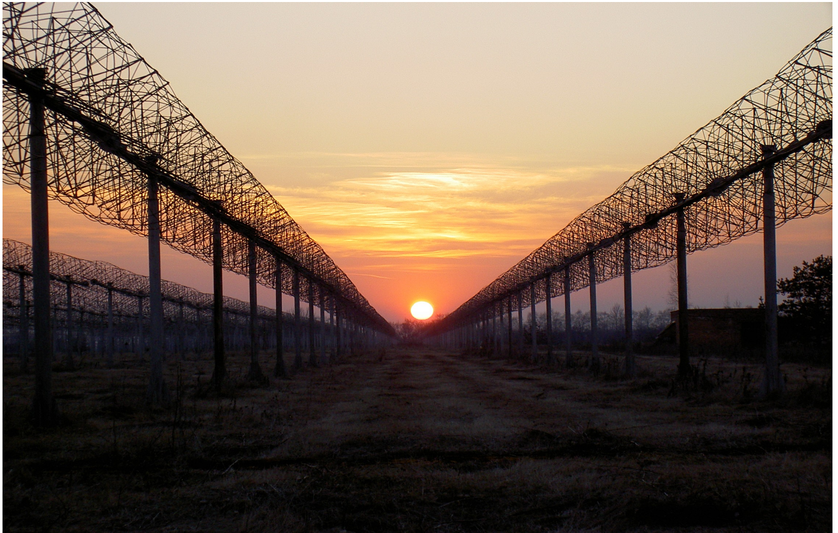
The UTR-2 radio telescope, E-W arm (900m×60m)
